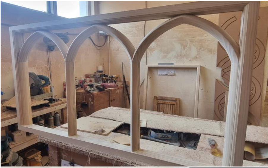
New window being made for St Nicholas Church.
